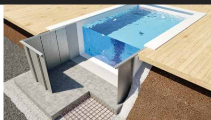
Steel panel construction
